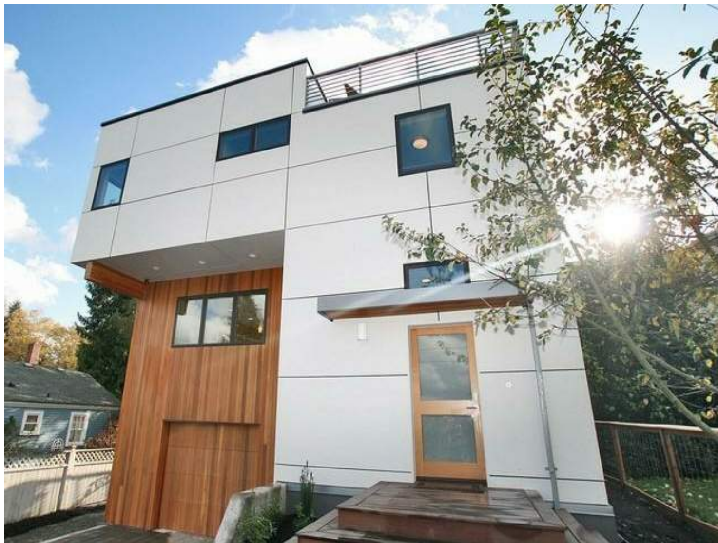
HARDIE REVEAL PANEL (SMOOTH) W/ PAINTED EXP. FASTENERS; COLOR ARCTIC WHITE (#4)
