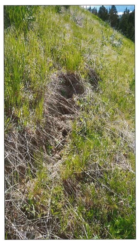
Photo 3: Looking at the tension crack in the fill slope at the rear of one of the un-developed lots to the southwest of the pump station.
