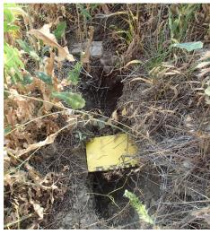
Photos 6 & 7: Open tension cracks on slope.
