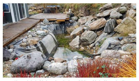
Photo 4: Setback of the house from the slope and failure of the boulder-stack wall.
