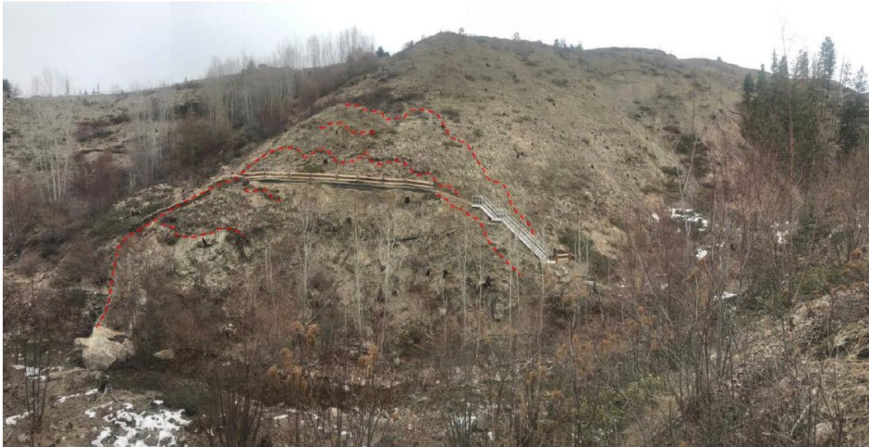
Figure 1: Tension Cracks Observed at Canyon Falls Trail Landslide
