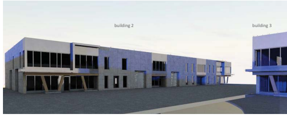
View from Optic Court
