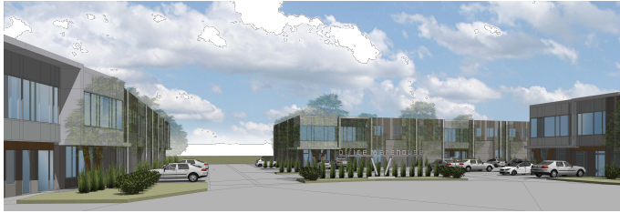
View from Optic Court
