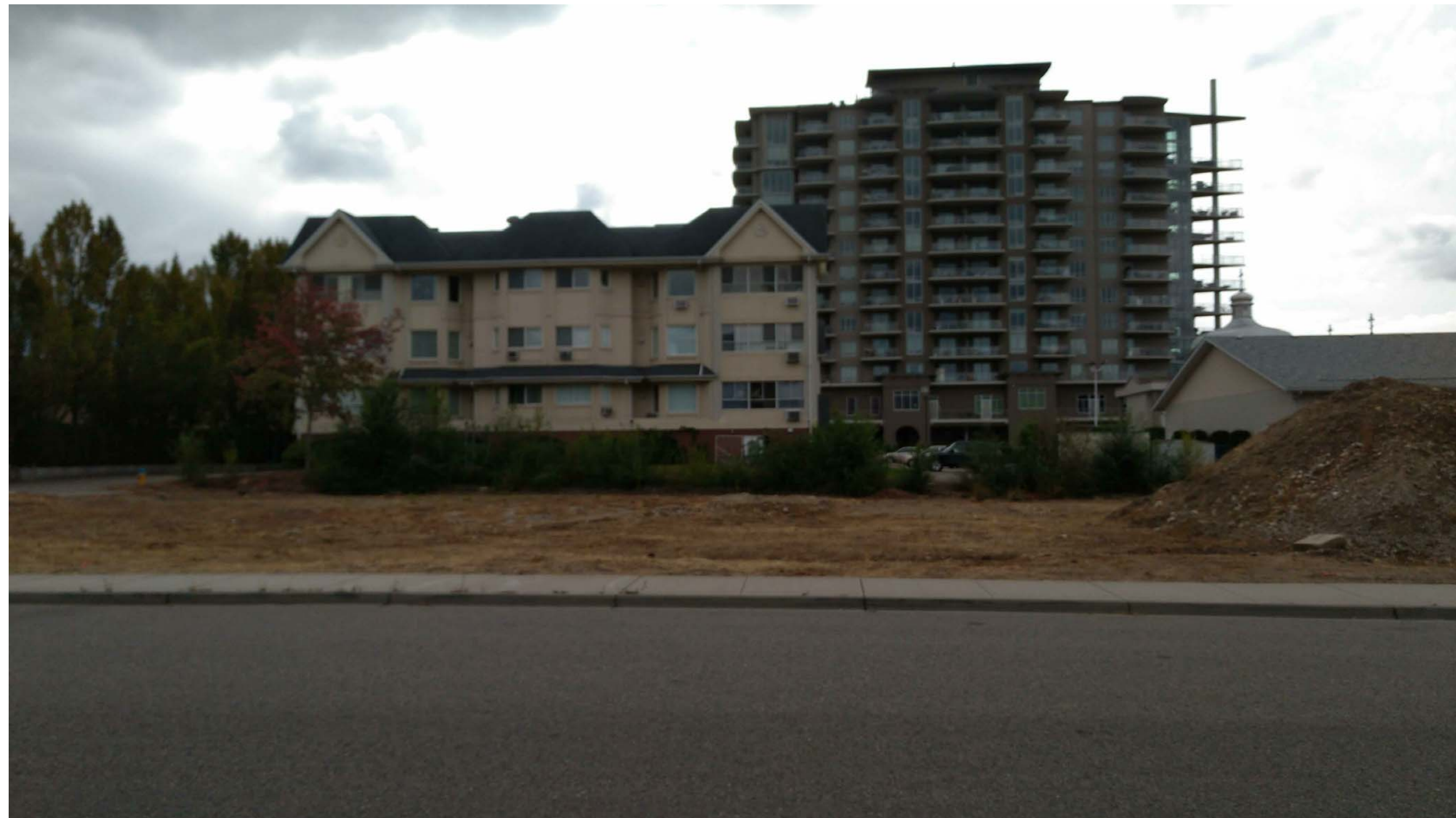
VIEW FROM AGASSIZ ROAD C
