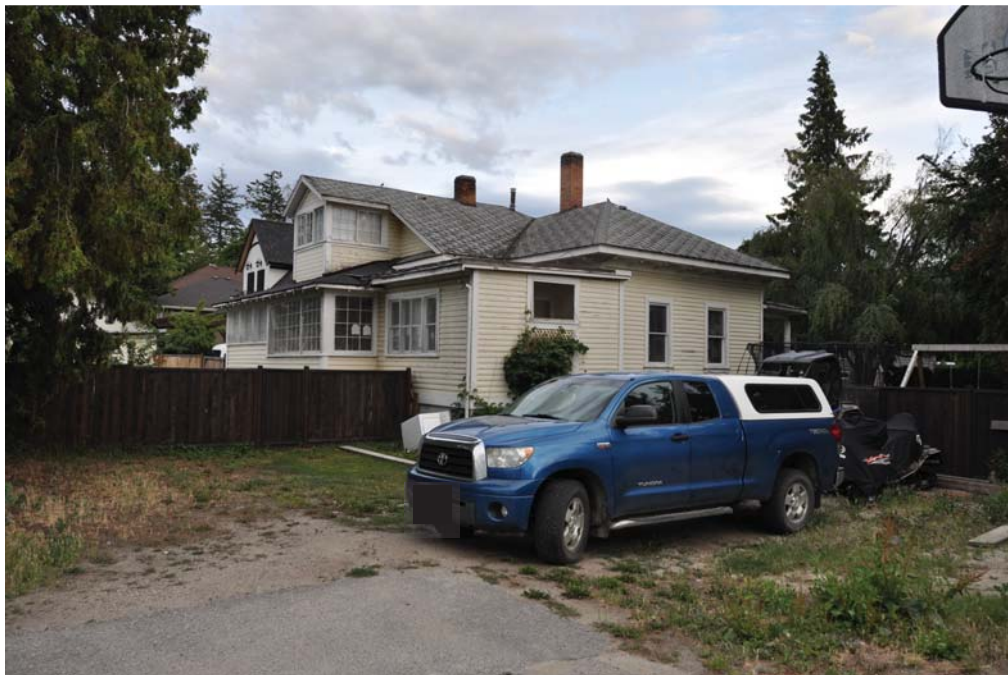
Photo 4. Rear view of Smith residence from northwest (Doryan Street). Flat roof bedroom add-on shown in foreground, with converted porch to the left of the bedroom.
