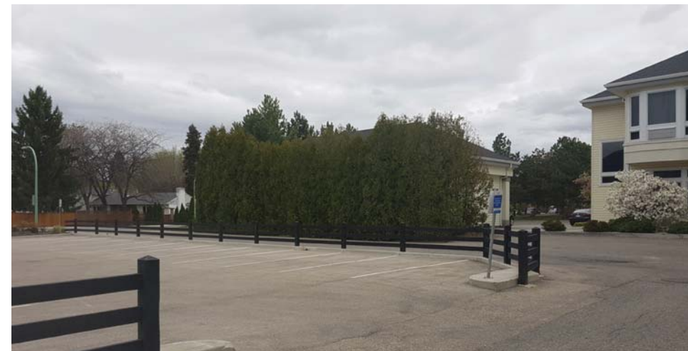
Photo 3 & 4 show existing curb, fence, and asphalt of east side of existing parking lot intended to be retained, resurfaced and repainted - refer to drawing A2.01
