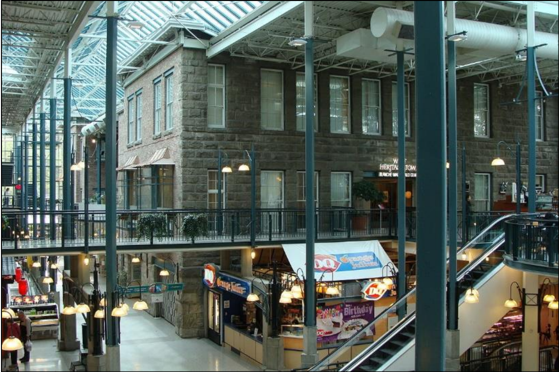
Fig. 1: City Square Shopping Centre, Vancouver, BC. Two 19 th century stone buildings were incorporated and enclosed in the design of a new commercial, retail and office space. Completed in 1989 with a $32,500,000 budget. (Source: Merrick Architecture)
