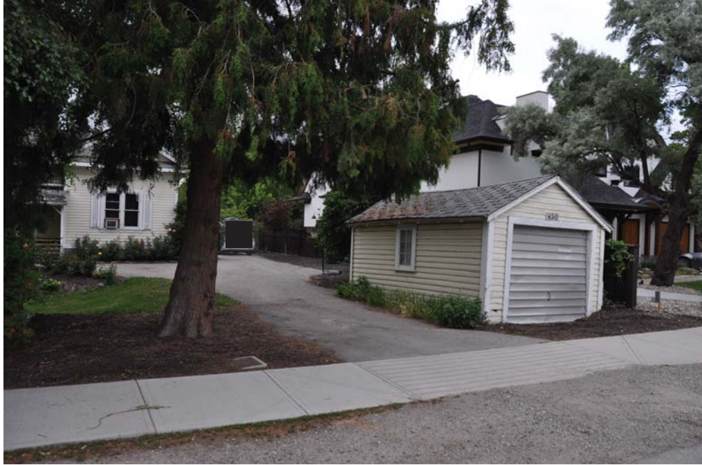
Photo 7. Early garage in southeast corner of property facing Cadder Avenue. Will be re-clad with same siding as the residence.
