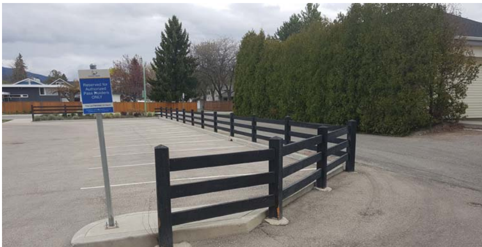
Photo 3 & 4 show existing curb, fence, and asphalt of east side of existing parking lot intended to be retained, resurfaced and repainted - refer to drawing A2.01
