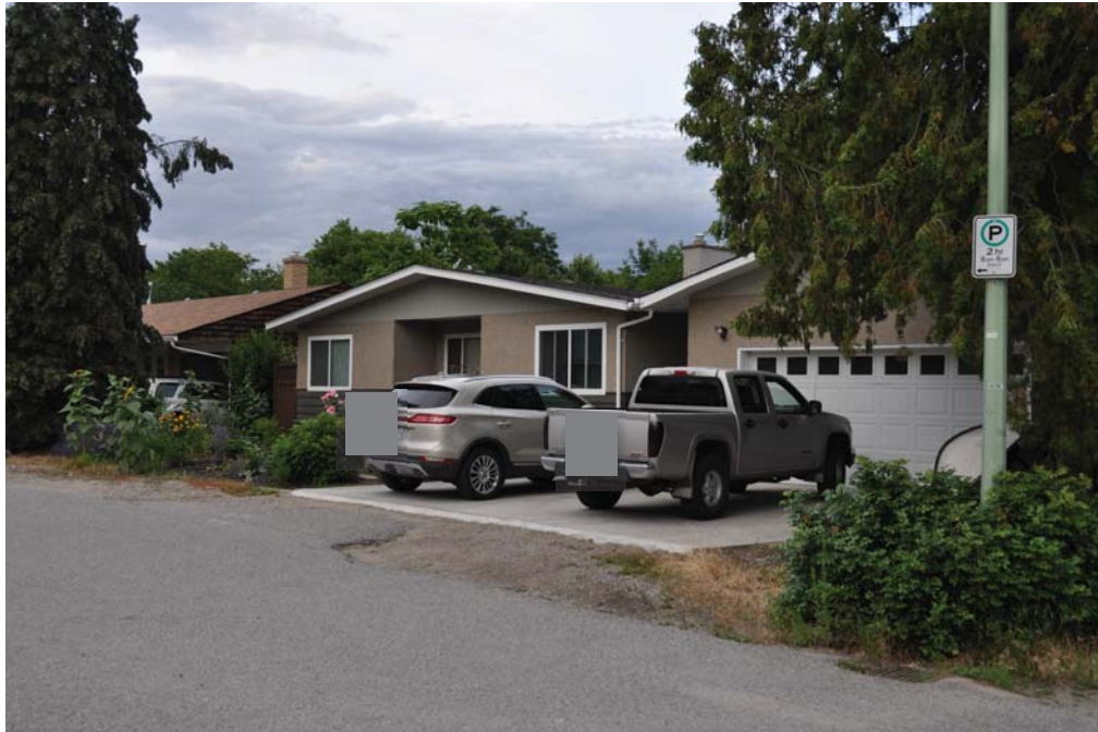
Photo 15. Neighbor's residence directly to the north, accessed from Doryan Street.
