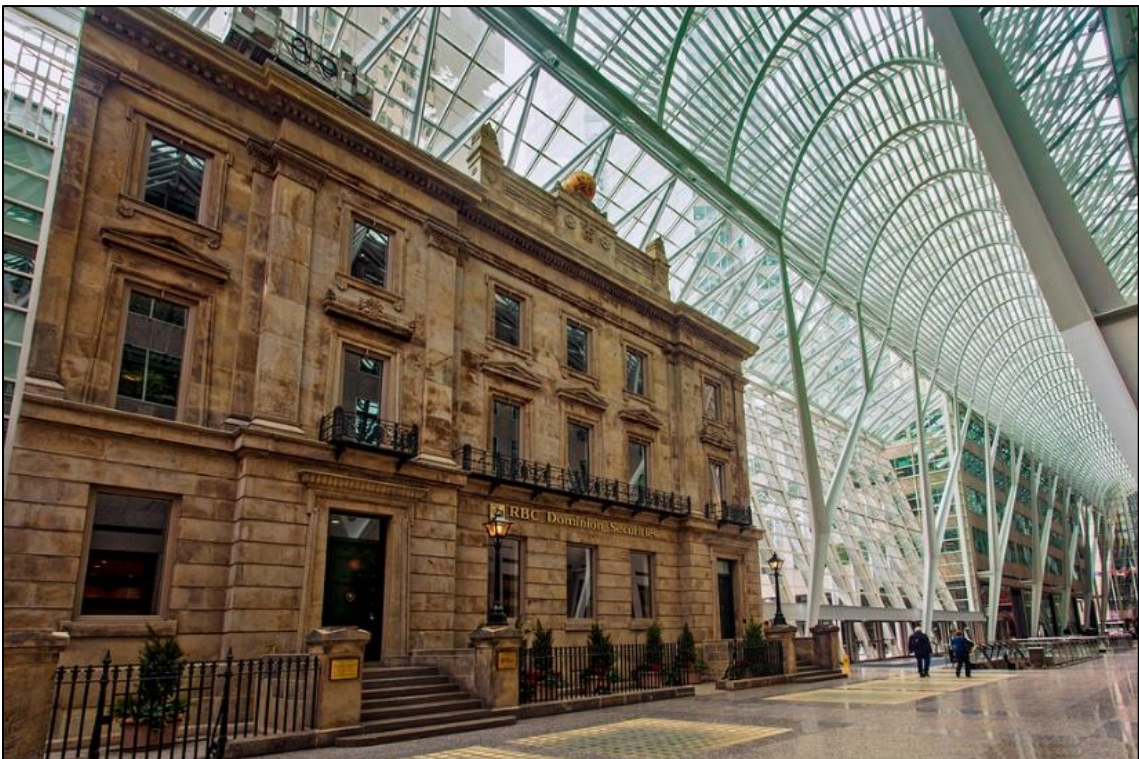
Fig. 2: Brookfield Place, the Allen Lambert Galleria, ON. A pedestrian thoroughfare incorporating the façades of eleven 19 th century commercial heritage buildings in its new design. Completed in 1992 for an undisclosed amount. (Source: John Dorosiewicz)
