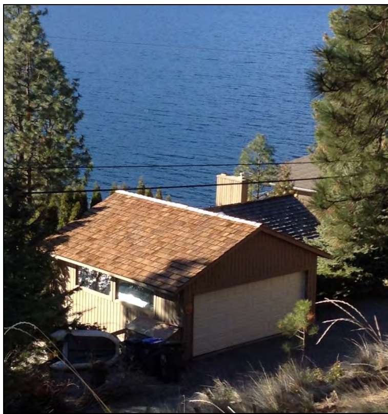
Figure 13. New shake roofing in the North Clifton neighbourhood. Mature pine trees adjacent will likely contribute additional combustible material to the roof, if allowed to accumulate.
