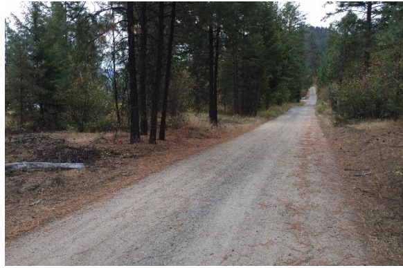
Current Condition of Shanks Road – South View
